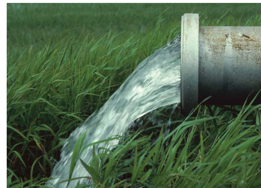
(Top photo) A rains garden is located in a parking lot instead of conventional plant islands which helps clean and replenish the water table. (Bottom photo) Shows water used for landscape and turf. IMU currently only waters a very small portion of their turf which could be turned off completely to reduce water use on site.
