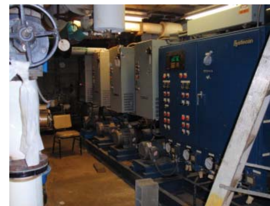
Images above depict the primary mechanical room of the IMU. The mechanical room houses the steam and chilled water service entries, pumps, controllers, and heat exchangers.
