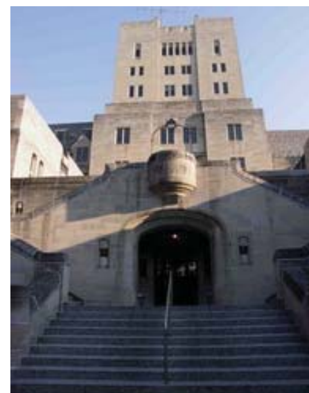
North side stairs to "front entrance" from 7th Street. Photo credit: IU Photography
