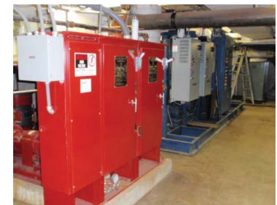
Images above depict the primary mechanical room of the IMU. The mechanical room houses the steam and chilled water service entries, pumps, controllers, and heat exchangers.
